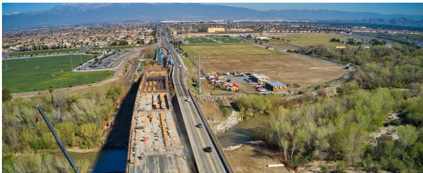
North facing view of the western span of the new bridge. Crews will be placing concrete on the deck of one segment and the stem and soffit of another segment this month.
