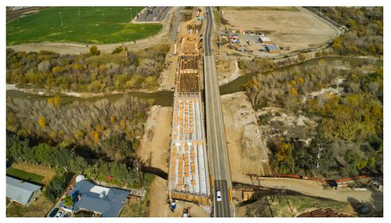
A north-looking view of the temporary wooden structure for the new western bridge span on Hamner Avenue. Concrete will be placed in the second half of the bridge interior, followed by more concrete placement on the bridge deck in early 2022. This bridge span is expected to open in Spring 2022.
