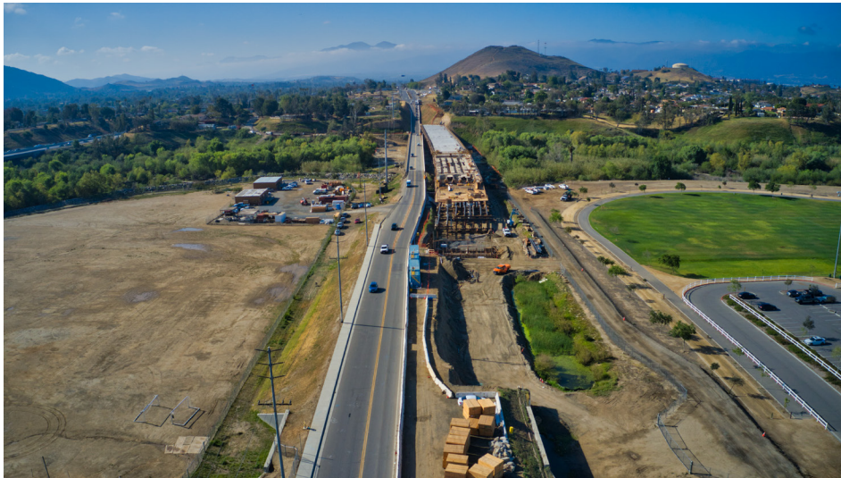
Looking southbound at work on the western span of the new bridge.
