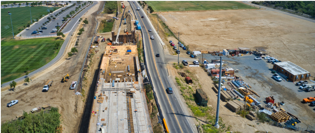
Looking north above Hamner Avenue, crews are working at different segments on the western span bridge structure.
