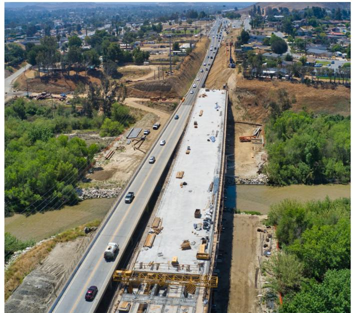
Crews making progress and working towards the next concrete placement for the next segment of the new western bridge span. The top portion of the structure shows the current state of the bridge deck, the bottom section shows the current state of the "interior" or the stem and soffit of the bridge.
