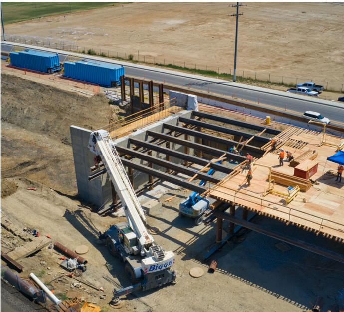
Carpenters and iron workers constructing the next segment of the new western bridge span. They are working to connect the bridge support abutment wall (left side) with the current bridge structure (right side).
